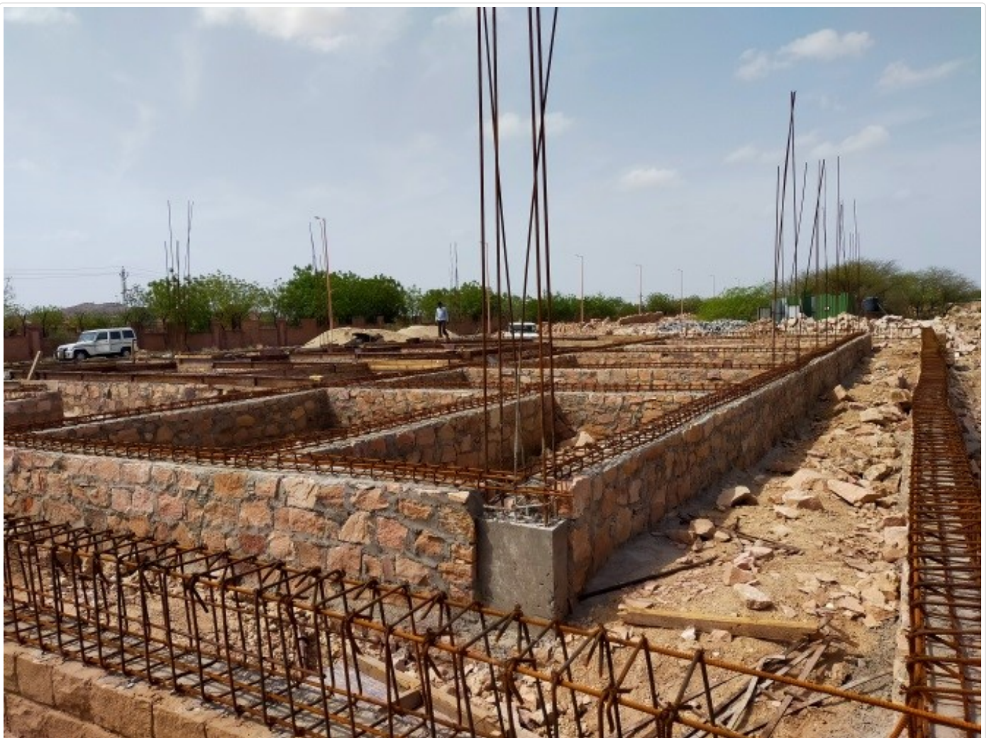
The site is under construction.
